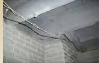
Install the loop wire above the ceiling, around the room or under the floor. The wire must form a continuous loop around the listening area. Do not install the loop wire close to and parallel with data lines, telephone, audio, or video cables. Avoid areas that include dynamic microphones.
